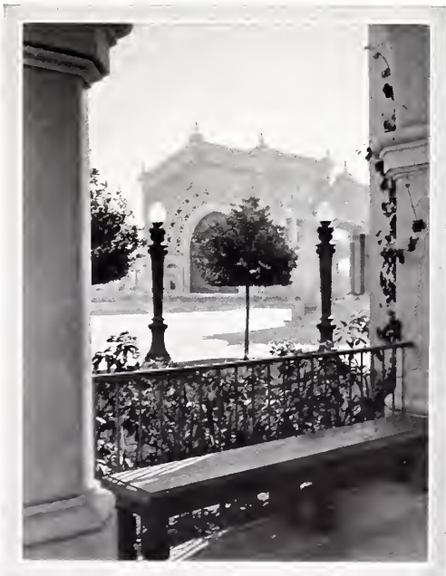
VISTA OF THE PIPE-ORGAN H. A. ERICKSON
